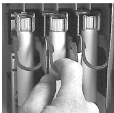
Built-In Fuse Pullers (NEMA 12 and 4X 30–200A Only)
